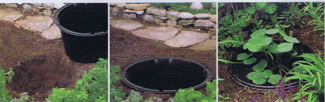
Above, left to right: Dig a hole to accommodate your tub; level the bottom of the hole with a 1-inch layer of sand. Sink the tub so the rim sits approximately at ground level. Set a container-planted specimen in the tub; cover with water. Conceal the tub rim with layers of stone.
